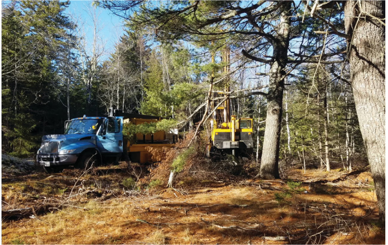
Digging test wells at Jones Marsh. IHT PHOTO
